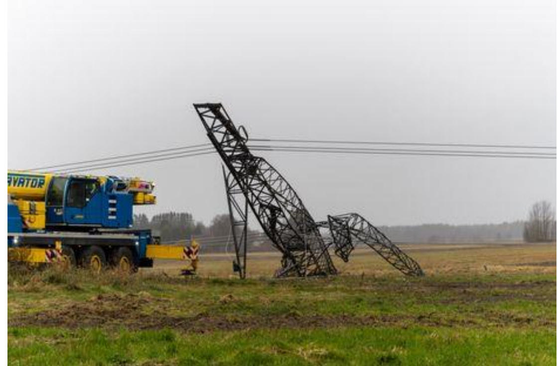
Hurricane knocked down a 400 kV pole in Eura, Finland (!)
